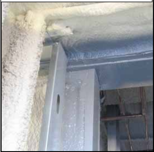
Complex window head at insulated overhang.
