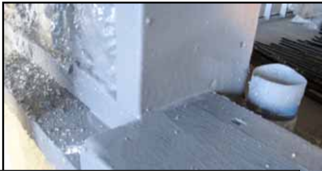
LAM allows air and watertight connections to difficult substrates at this expansion joint that occurs where a school addition meets existing brick construction.
